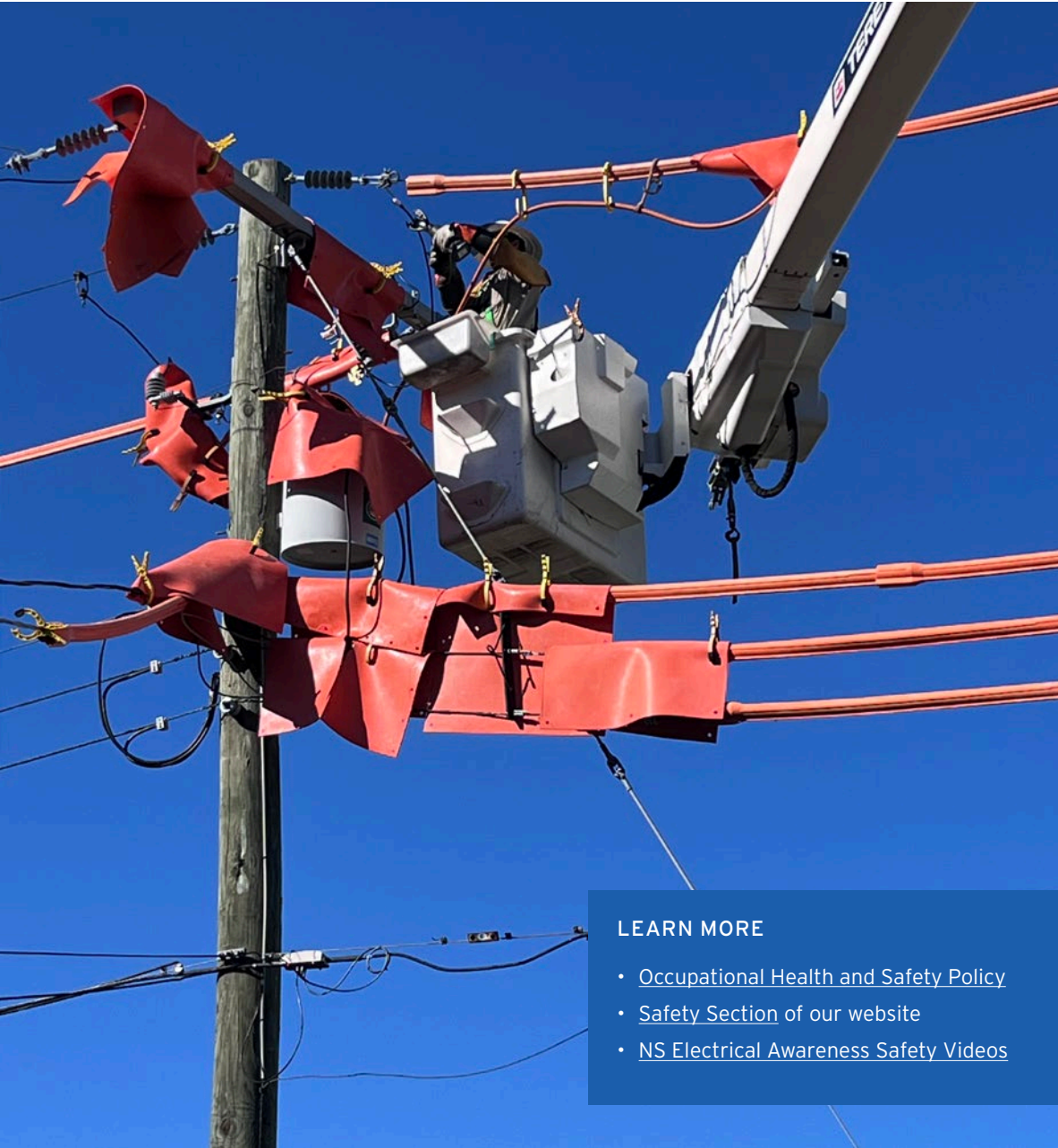
A power line technician working on Tampa Electric power lines with protective cover-up applied.
